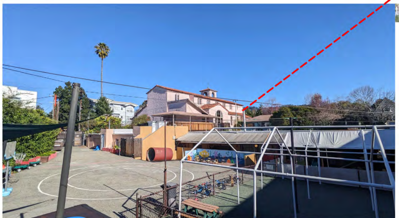
VIEW FROM SOUTHWEST CORNER OF SITE- EVERYTHING TO BE DEMOLISHED
