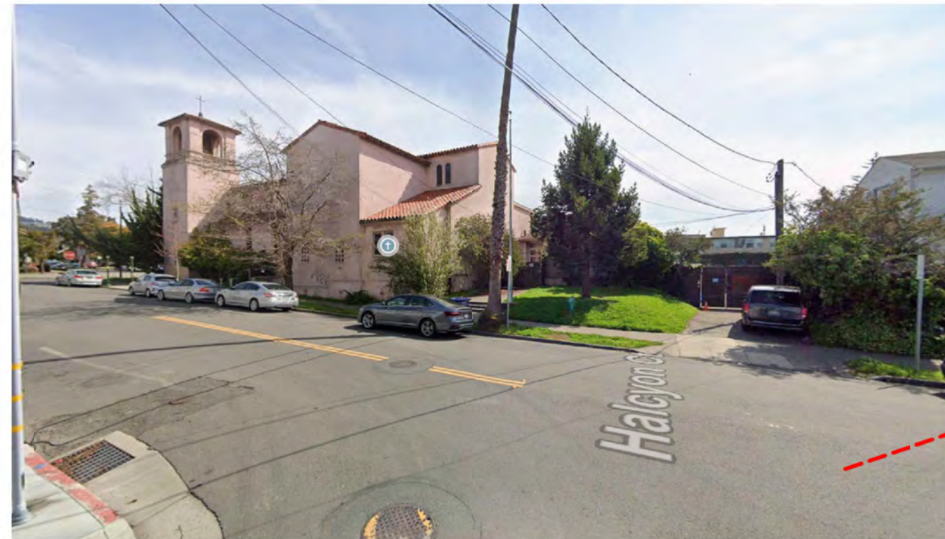
VIEW OF PROJECT SITE FROM HALYCON CT.- STREET
