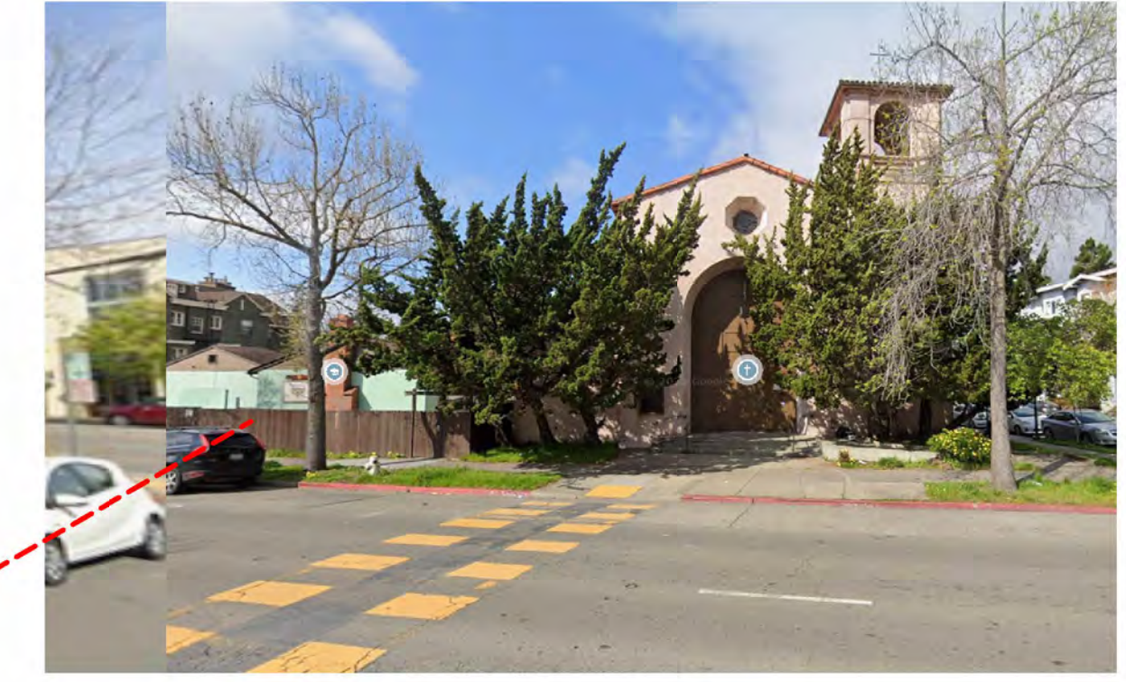
VIEW OF PROJECT SITE FROM CORNER OF PRINCE ST. & TELEGRAPH AVE.
